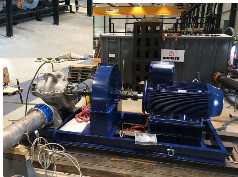
Open-pit testbed 300 bb type of pumps
